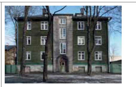
Protection of body A fire-resistant core was prescribed for stairways of Tallinn timber houses, to protect the bodies of those who inhabited them. The earliest vertical form was reproduced on a city-wide scale. A mausoleum protects and signifies a body that has left, it has the doors and stairs and windows. Location Tallinn Author Karl Treumann Year 1934
